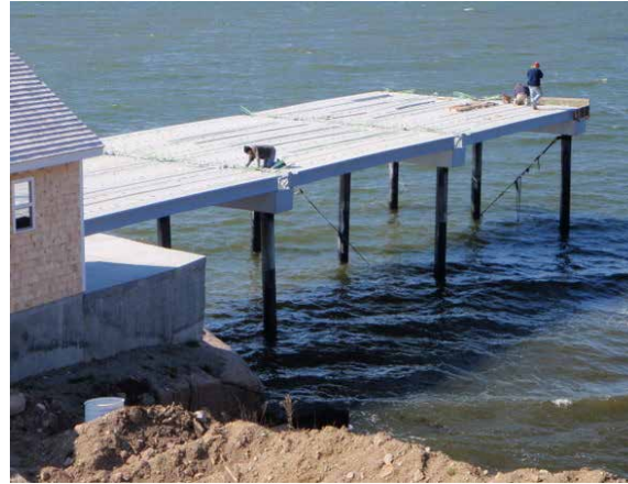
Composite decks and floating docks for Downeast Institute [Harbor Technologies, Brunswick, ME]
