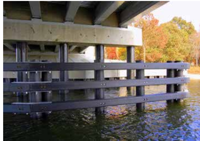
Two 56'x11'x4' cruise ship stand-off floats for Cruise Terminals of America, Seattle, WA (left) and Bridge Fender with HarborPiles on Beach Boulevard Bridge over Forked River, NJ (right) [Harbor Technologies, Brunswick, ME]
