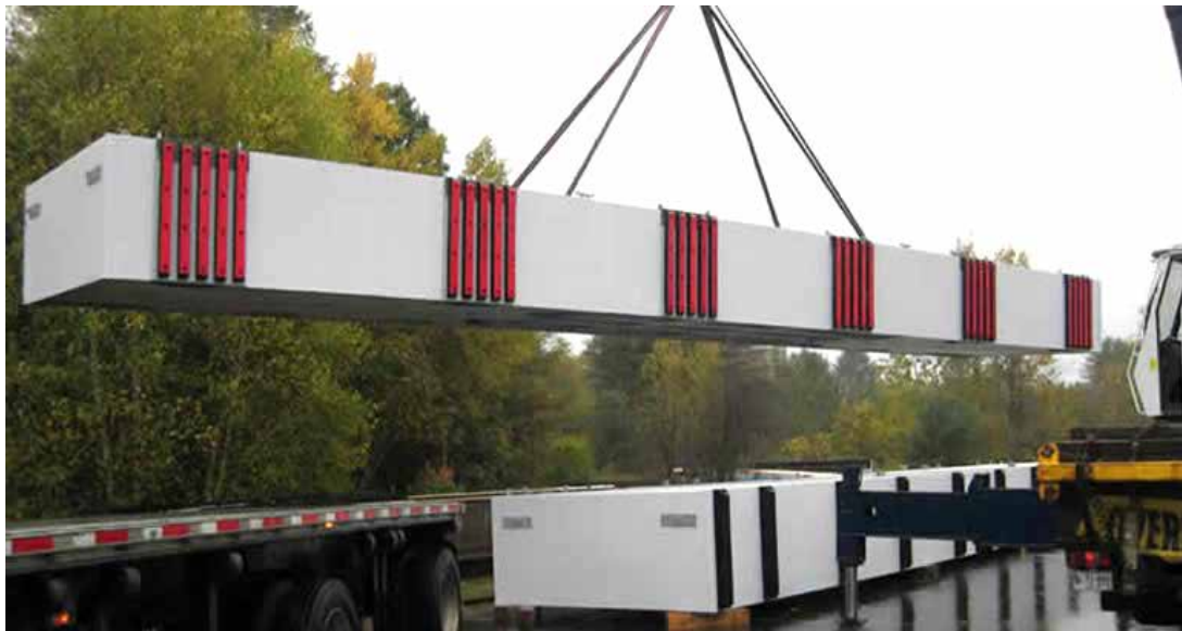
Two 56'x11'x4' cruise ship stand-off floats for Cruise Terminals of America, Seattle, WA (left) and Bridge Fender with HarborPiles on Beach Boulevard Bridge over Forked River, NJ (right) [Harbor Technologies, Brunswick, ME]
