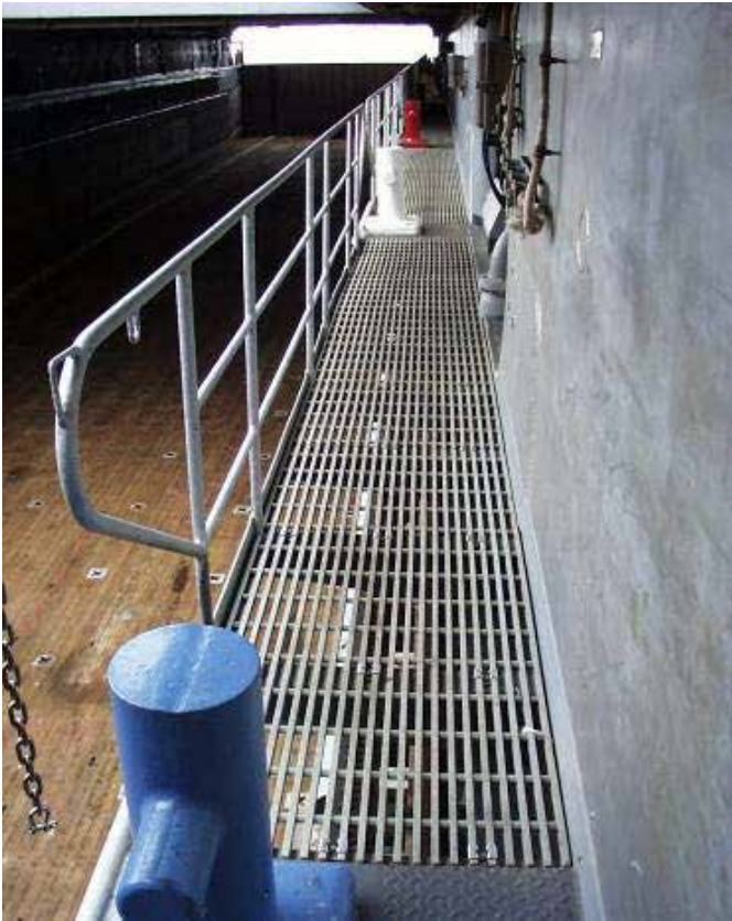
LSD Wing Wall
