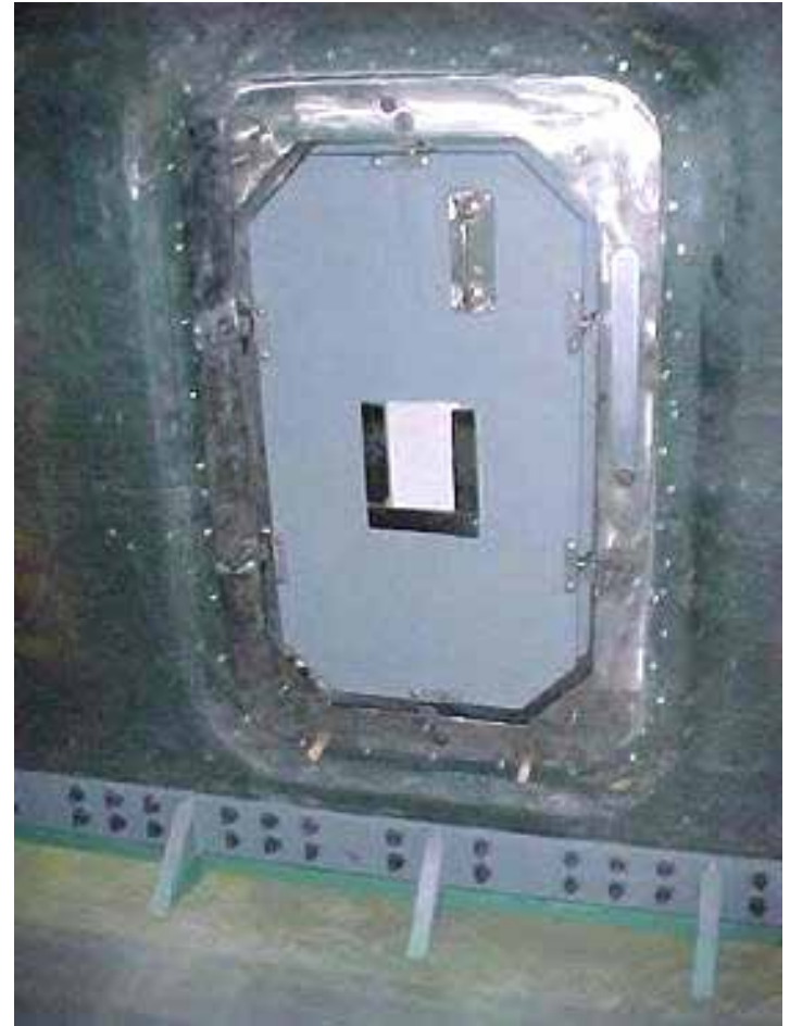
E-Glass/Vinyl Ester-Paneled Door Built by Ingalls used in ManTech Topside Project
