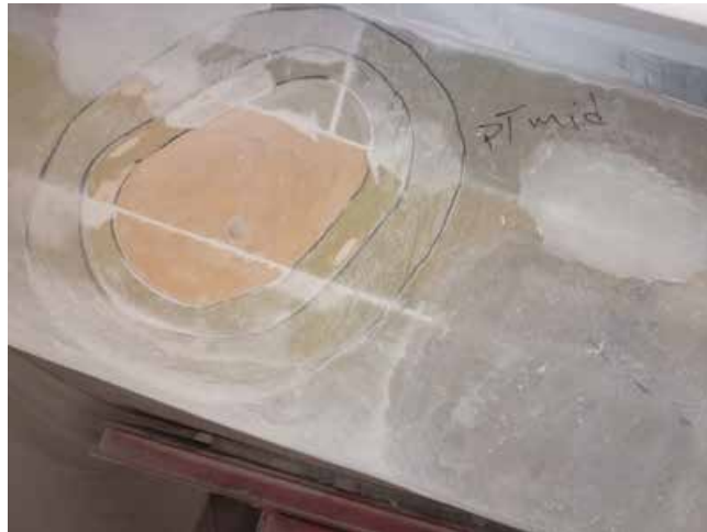
Mark area for repair reinforcements
