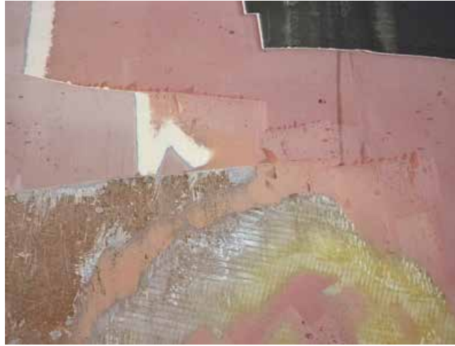
Multiple layers of existing fairing
