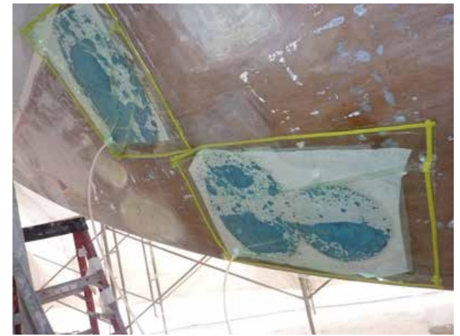
Using vacuum bags to consolidate repairs
