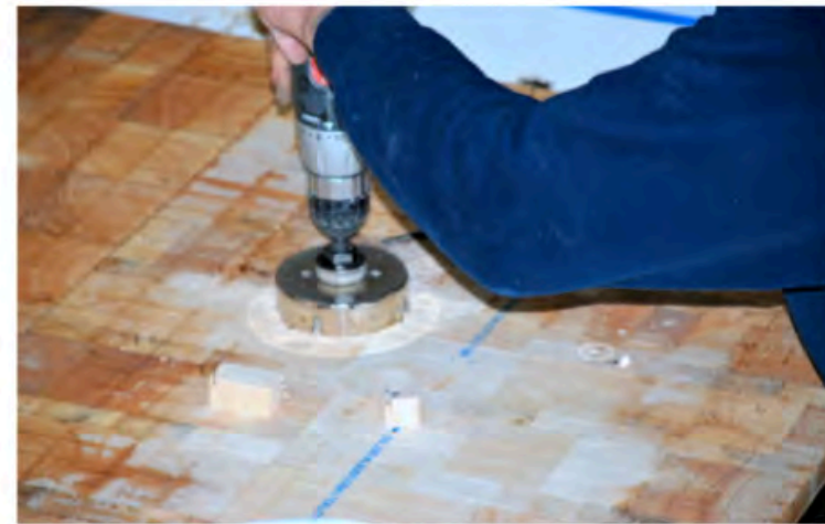
Hole saw is used to create a 1/8 inch deep void for water to be encapsulated
