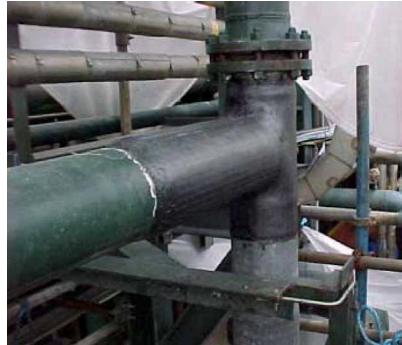
Carbon fiber repair of 14 inch tee joint on a seawater return header
