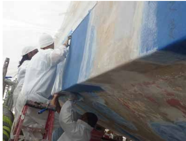
Waterline lamination in progress
