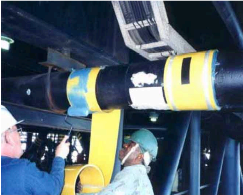
'Clockspring' repair to an externally corroded pipe
