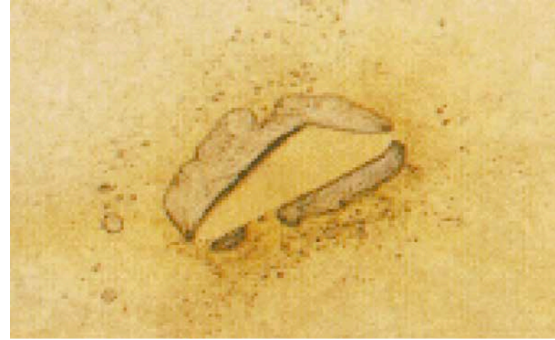
Resin pocket Apparent accumulation of excess resin in a small localized area
