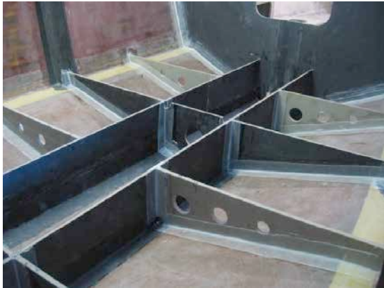
Structure Showing Framing with Carbon Skins over PVC Core
