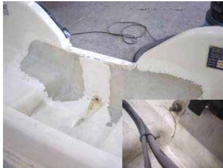
A repaired stress crack as shown in inset photo
