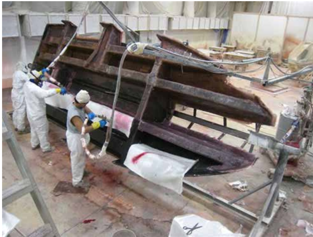
Reinforcement is Added to Structural Grid
