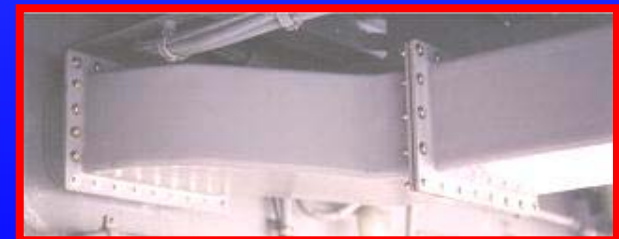
Prototype Composite Ventilation Duct System Built by Boeing and Structural Composites Installed on the USS Samuel B. Roberts , FFG-58
