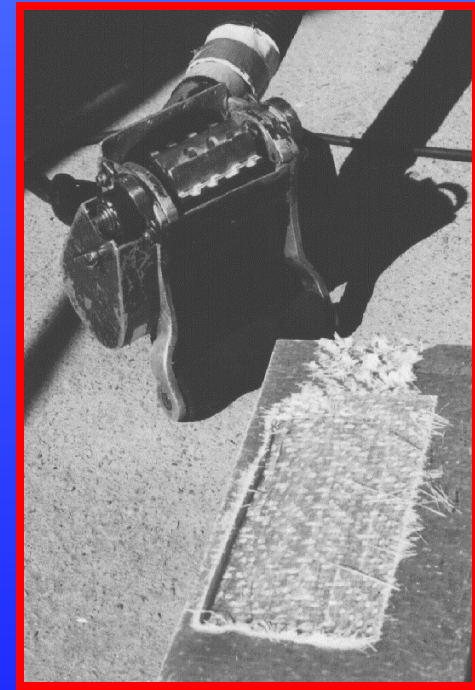
Laminate Peeler used to Repair Severe Blister Damage
