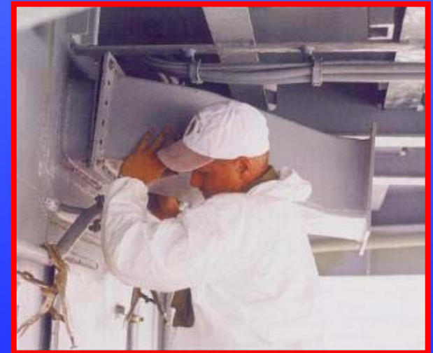
Prototype Composite Ventilation Duct System Built by Boeing and Structural Composites Installed on the USS Samuel B. Roberts , FFG-58
