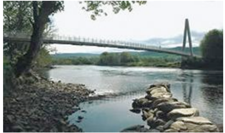
Composite footbridge built in Scotland in 1990 (top) and large carbon fiber beams from Strongwell (bottom)
