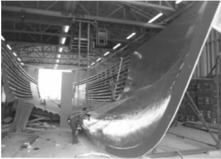
Figure 5-6 Batten Construction of Female Mold at Westport Shipyard [Westport photo]
