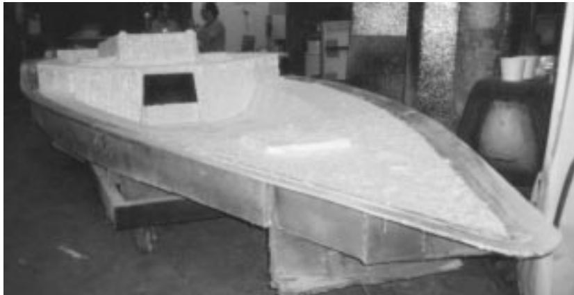
Figure 5-35 Dry Reinforcement In-Place for SCRIMP sm Process [Mosher, TPI]
