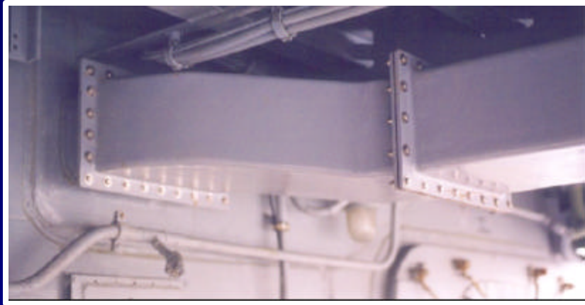
Composite Ventilation Ducts on FFG 58 built by Structural Composites
