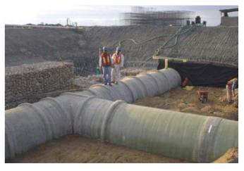
Composite pipe up to 4 meters in diameter has been manufactured for water handling. Shown here is an LNG re-gasification seawater intake pipe.
