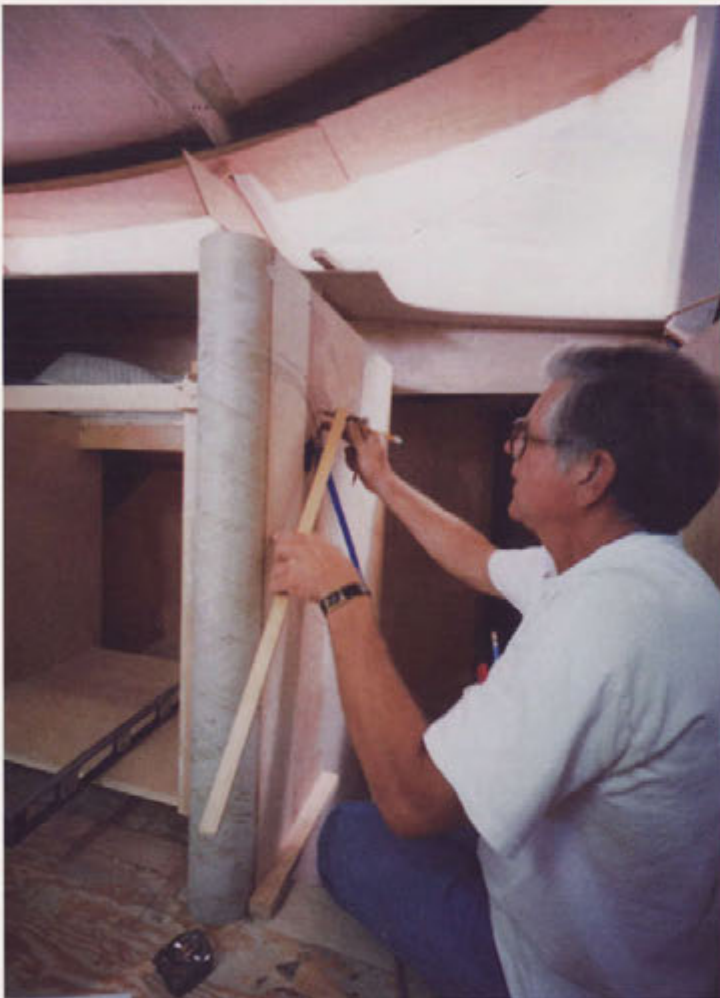
Master carpenter Terry Berton scribes the handrail for the main companionway. Berton was responsible for the fabrication of all the custom joinery that distinguishes TEEL's interior.
