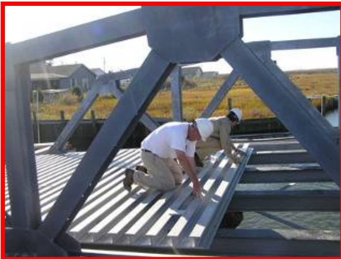
Installation of ZellComp composite bridge decking in Bradford VT (top) and Tangier, VA (bottom)
