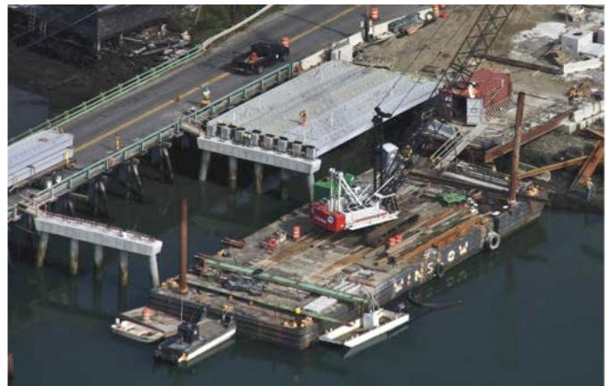
This 32-foot-wide, eight-span, 540-foot long composite bridge uses hybrid composite beams manufactured by Harbor Technologies.
