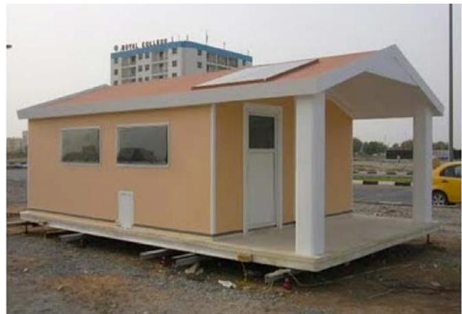
InovaTec composite houses are assembled in 25% of the time needed for conventional construction, don't require cranes, resist earthquakes and CAT 5 hurricanes and are insulated to R 24 values.
