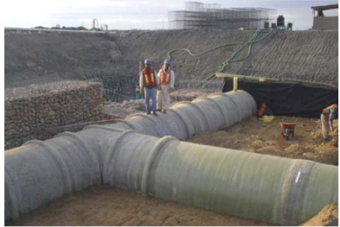
Composite pipe up to 4 meters in diameter has been manufactured for water handling. Shown here is an LNG re-gasification seawater intake pipe.
